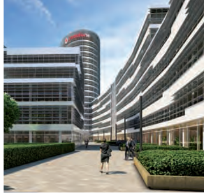
Links: Airgate in der Airport City; daneben: Vodafone Campus Düsseldorf.
