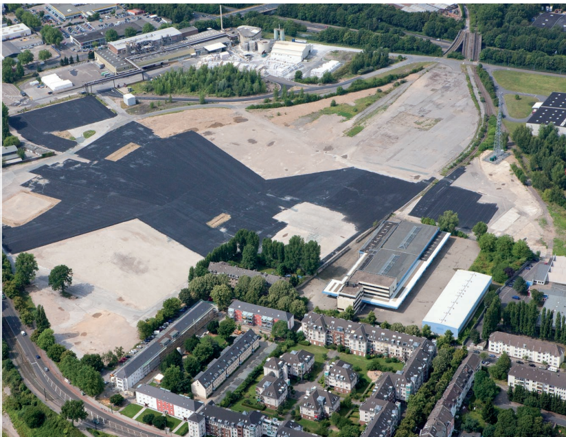
16 ha in Benrath awaiting new tenants: the planned SEGRO business park.
